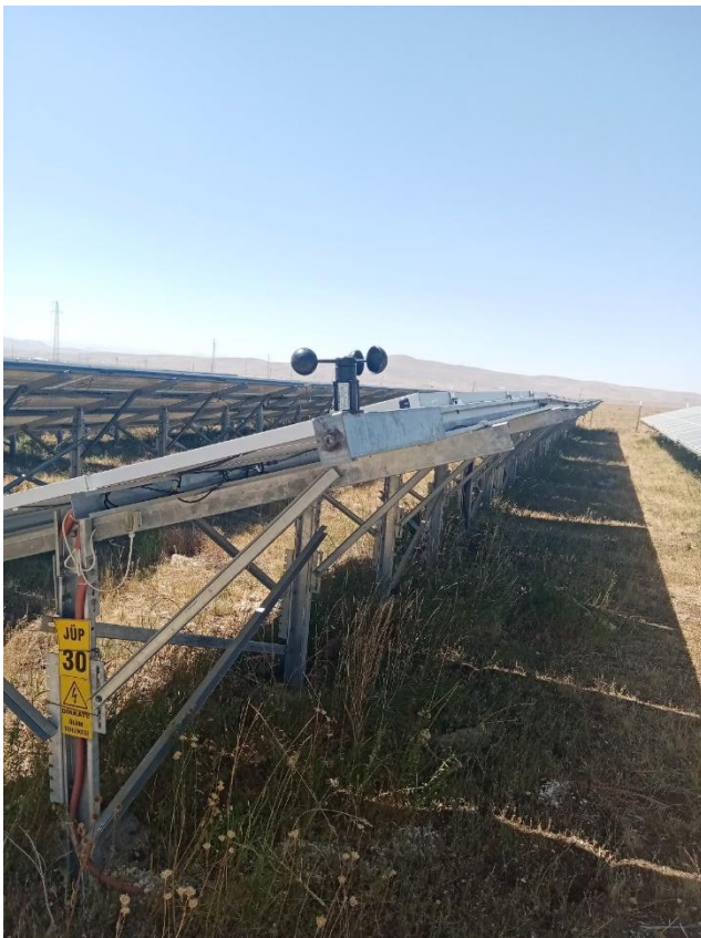
Figure 2: The weather station monitors the conditions in the module planes.
